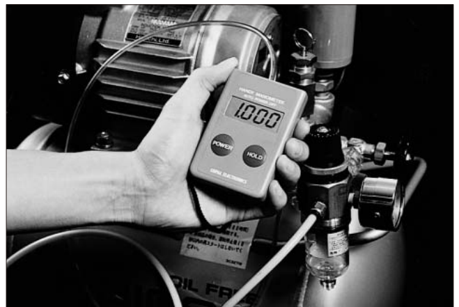
▲ Measurement of source pressure from a compressor.
